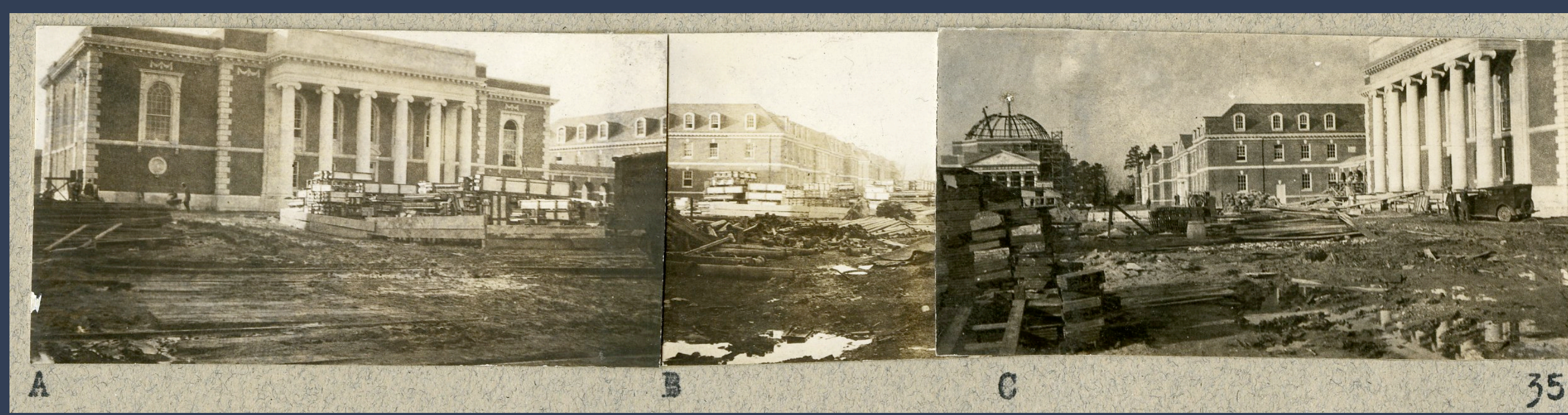
East Campus under construction. Olmsted Brother, 1920s. Olmsted Archives.
