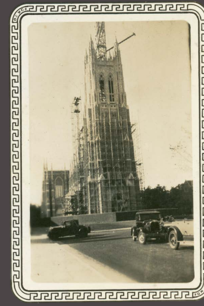
Duke Chapel construction nears completion. Photograph by former Duke student, Charles Wesley Clay, 1930s. Duke University Archives.
